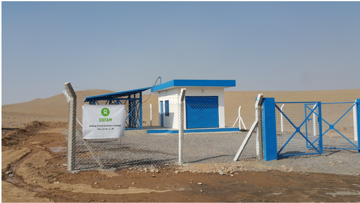
New borehole being drilled in Debaga, Iraq. Photo: Hassan Ibrahim/Oxfam
